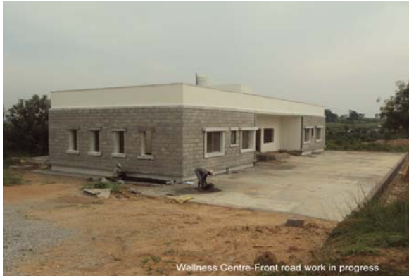
Wellness Centre-Front road work in progress
