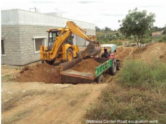
Wellness Center-Road excavation work
